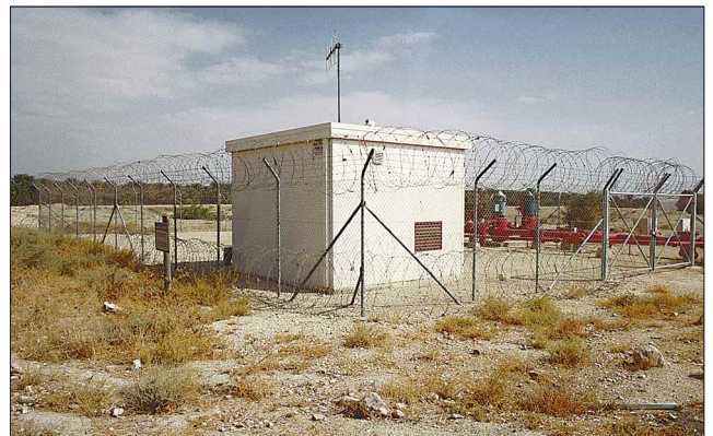
Fenced enclosure and wellhouse, Jordan Valley, north of Jericho
